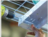
**STEP 4:** Connect power from building to quick disconnect on retrofit kit. Bring retrofit kit up to fixture frame.
