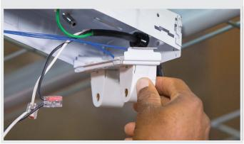
**STEP 3:** Break apart the 1-piece mounting bracket kit into 3 individual pieces. Install a small bracket at each end of the fixture and the large bracket at the center of fixture (for 8' fixtures only). Bend the brackets over the fixture to fit the exact width and fasten them to the fixture with the provided tek screws.
